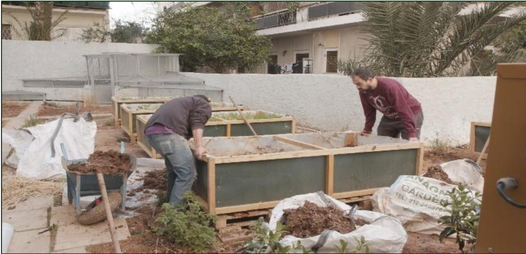
15. Figure: Photo of the Citizen Parking urban garden installation
