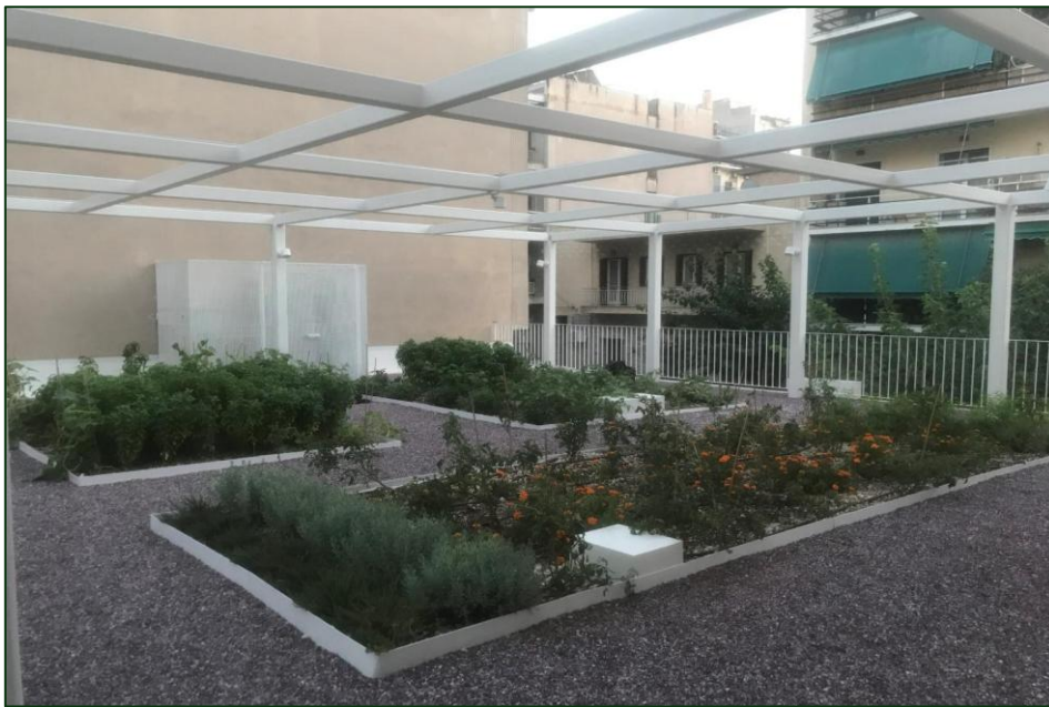
20. Figure: Green Stegi installation at Leontiou st. 47.8sm of planting on a 136sm terrace.
